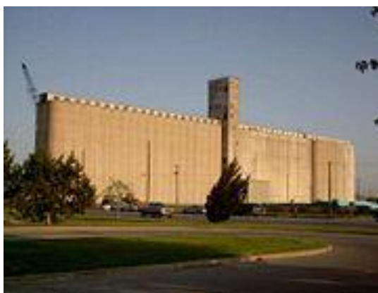
1928 Burrus Elevator (slipformed concrete silo construction in Lubbock, Texas. A steel reinforced concrete elevator with 123 silos shown just prior to demolition in 2004
